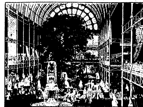
LIVING IN A GLASS SHELL in northern latitudes is comforting for tropical plants, but not for humans—without elaborate air conditioning. The visitors to Paxton's Great Exhibition hall were extremely grateful for the shade of the tall elms around which the glass vault had been assembled.
