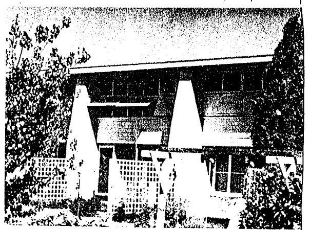
ADOBE BUTTRESSES AT CHANDLER FOR SHADE, PRIVACY
